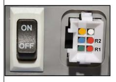
"Wake Up" the control by pressing the red and blue arrow keys. Set the water temperature setting not to exceed 120°F.
