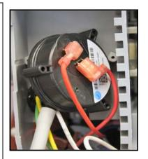
120V power is passed from the pressure switches to the control thru the red #1 wire on the blower Molex. This is the signal needed to energize the hot surface igniter.
