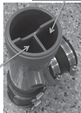
Blower Condensate Chamber
