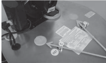
Anodes are located under caps.
