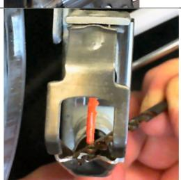
5. The igniter rod should be positioned in the bottom and middle of the saddle of the pilot hood as shown here.
