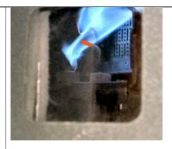
2. If not then remove burner/inner door assembly to gain access to the pilot assembly.
