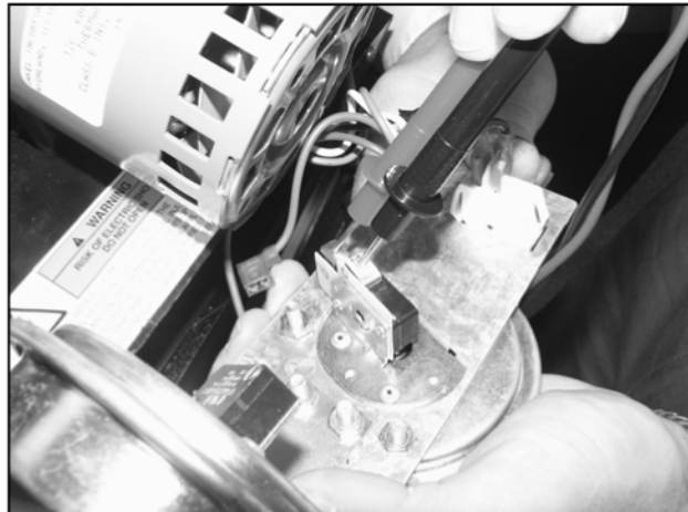
Blocked Inlet Switch FPD 251 Series
