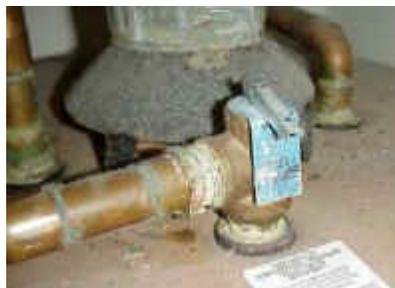
**Figure 1 - Typical installation of a Temperature/Pressure Relief (TPR) Valve on a gas water heater**
