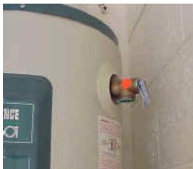
**Figure 3 - Missing TPR Valve discharge pipe**
