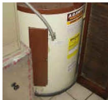
**Figure 5 - Inadequate Water Heater Spill Pan Sizing**
