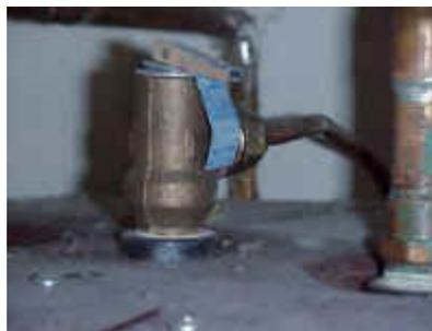
**Figure 2 - Improperly sized TPR discharge pipe**
