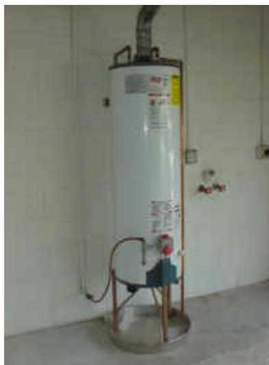
**Figure 4 - Improper Termination of Discharge Pipe.**
