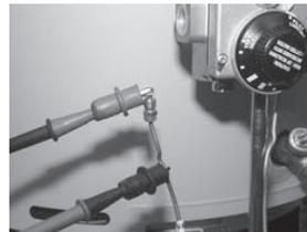
Step 3. Following the lighting instruction label on the heater, proceed to light the pilot and allow to operate for three minutes. **It will be necessary to hold the pilot button down continuously throughout this test.** A reading of 20 to 30 millivolts indicates good thermocouple output.
