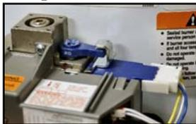
Listen for spark ignitor. Visually verify spark at the pilot electrode.
