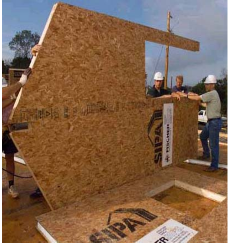
Figure 4 picture of the SIPS being installed in ZEH2
