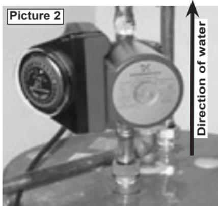
8. Plug the line cord of pump into a 115V outlet. Be sure to route the power cord so that it does not touch the exhaust vent piping of a gas or oil fired hot water heater.
