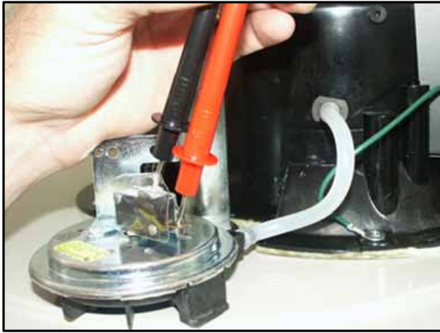
Continuity Test With Ohm Meter Power-Vent Residential Model
