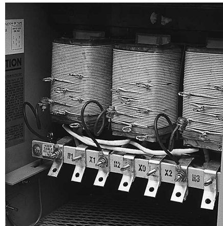
Wiring compartment for ventilated transformer
