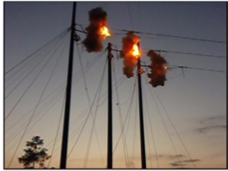
Figure 2.2-10 Multiple IMPLO® deadends being installed simultaneously.
