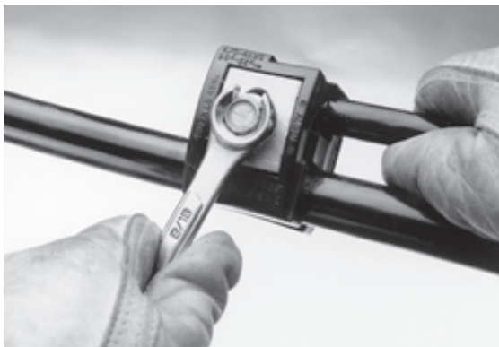
Figure 2.2-4 Installing an Insulation Piercing Connector
