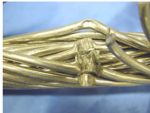
Damage from firearms
