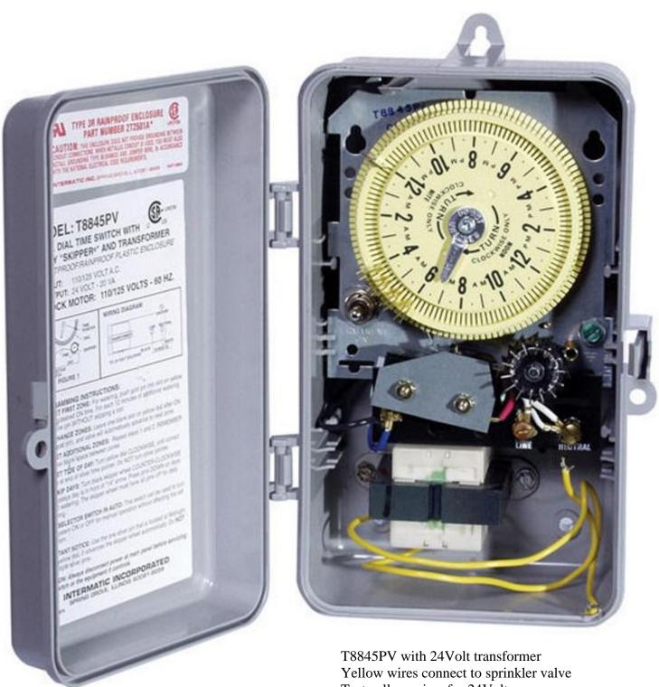
Yellow wires connect to sprinkler valve Test yellow wires for 24Volts Test Line and Neutral screw terminals for 120V Line is for black wire and Neutral is for white wire
